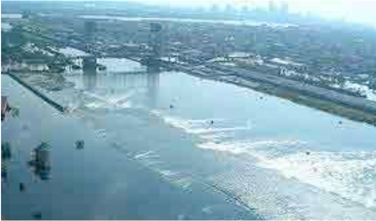
Figura 8.13 Levee failure following hurricane Katrina. Fuente: rice.edu. The Mississippi River breaching a levee in the aftermath of Hurricane Katrina.
