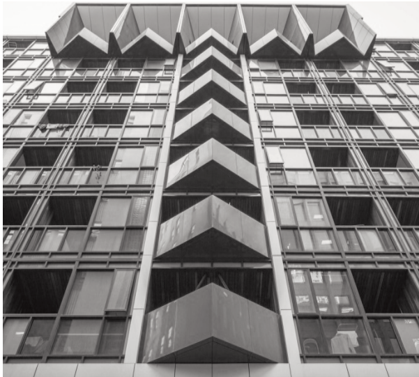
Figure 3-2. Little Hero Building (modular building in Melbourne, Australia).
