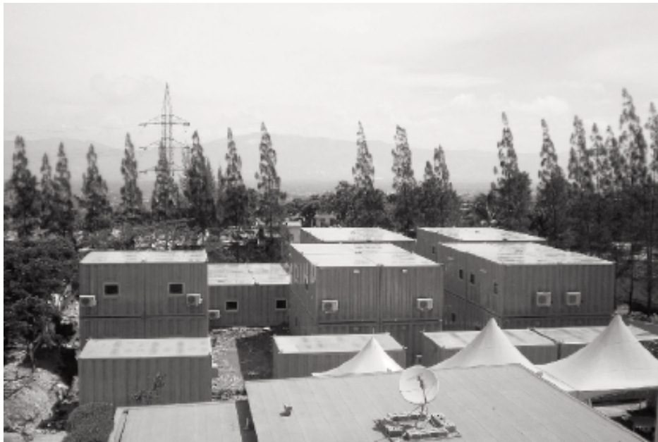
Figure 6. Modular housing units installed by the Canadian Embassy in Haiti (source: Sullivan Land Services, 2010).
