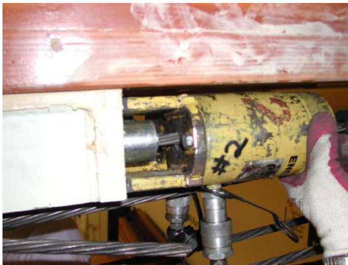
Figure 6. Cables are post-tensioned with hydraulic jack.
