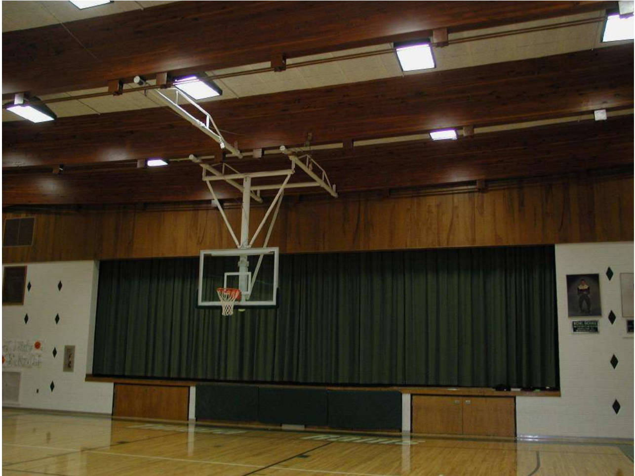
Figure 7. Completed repair/reinforcement of glulam girder beams.
