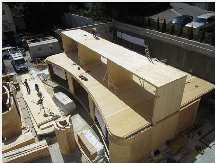
Fig. 6 - Prefabricated CLT elements are transported to the construction site and then assembled and erected manually: Waldorf School in Ljubljana, Slovenia built during 2009-2012.
