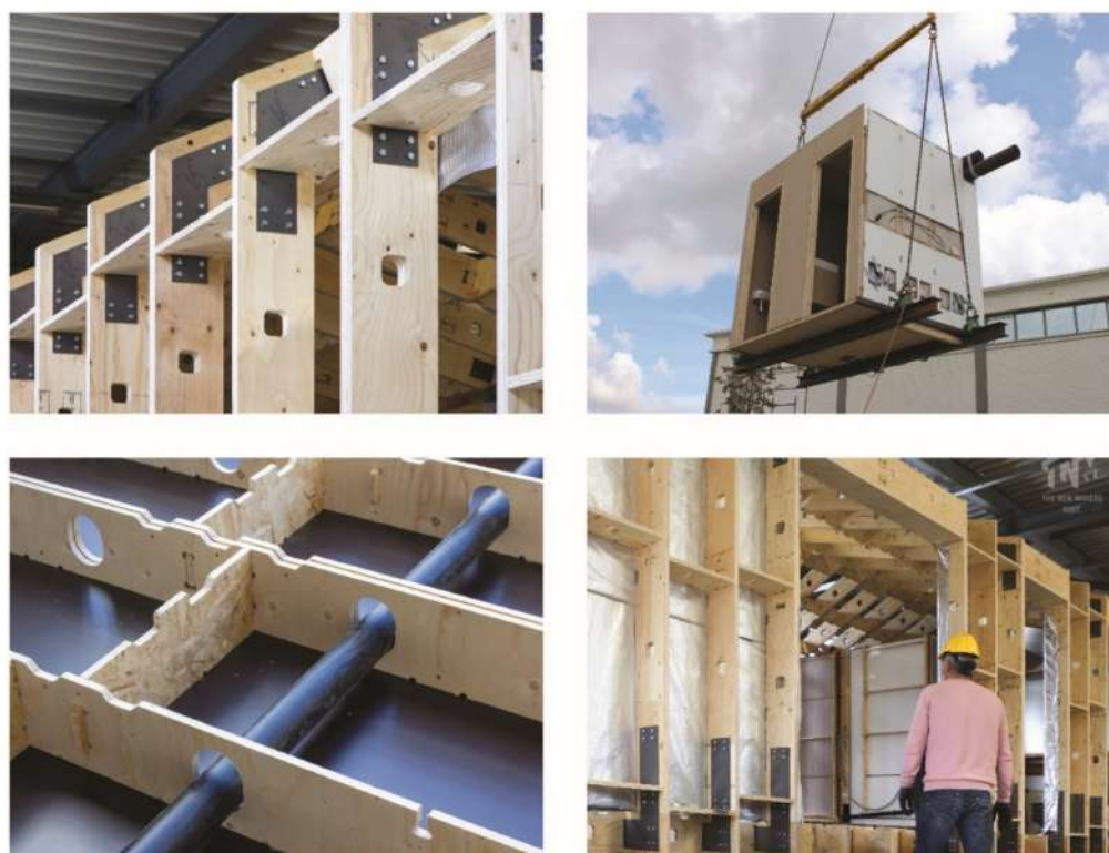
Figure 3. Uuthuske produced in the factory. Source: The New Makers.
