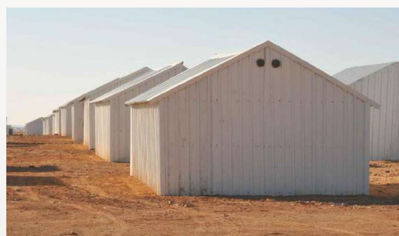
Transitional shelter: 2-4 years durability; steel structure and sheet metal, aluminum foam insulation
