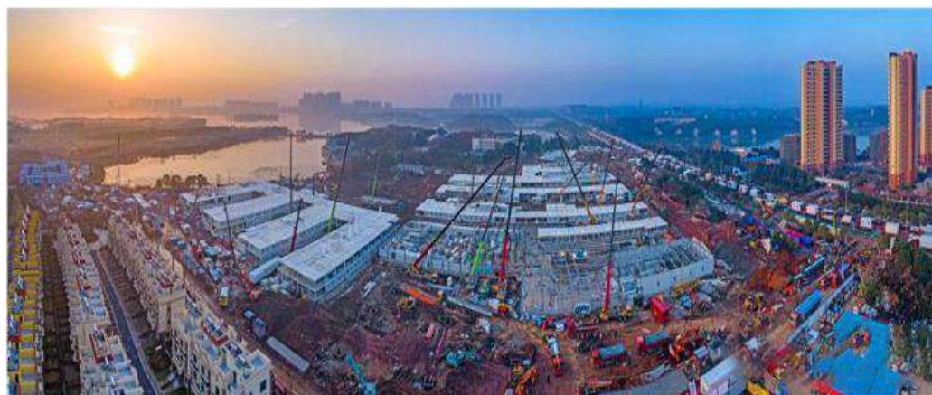
Figure 1. Wuhan Leishenshan Hospital [20].
