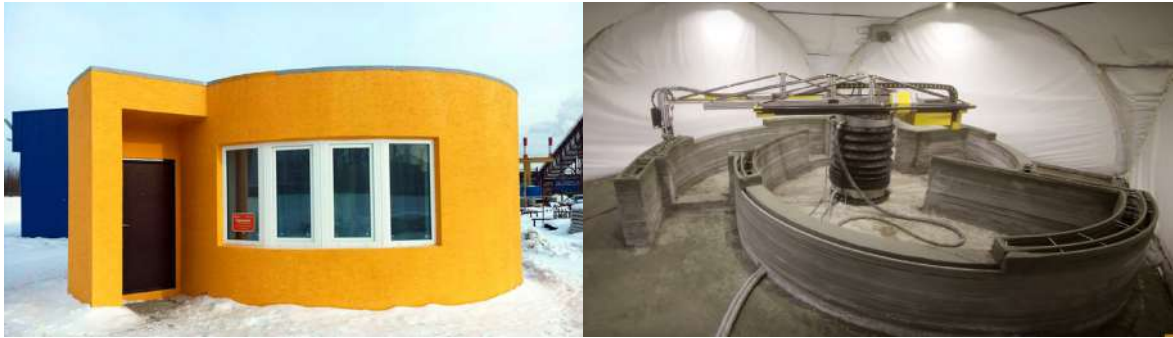
Fig. 2. (a) Front view of Apis Cor House in Russia;
