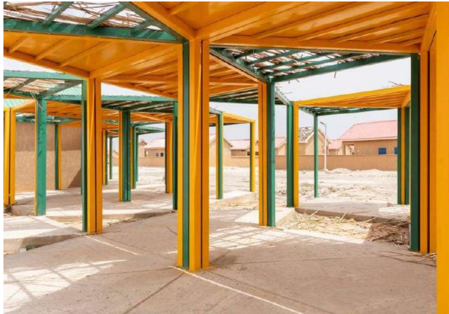
A colourful market pavilion was built at the centre of the village
