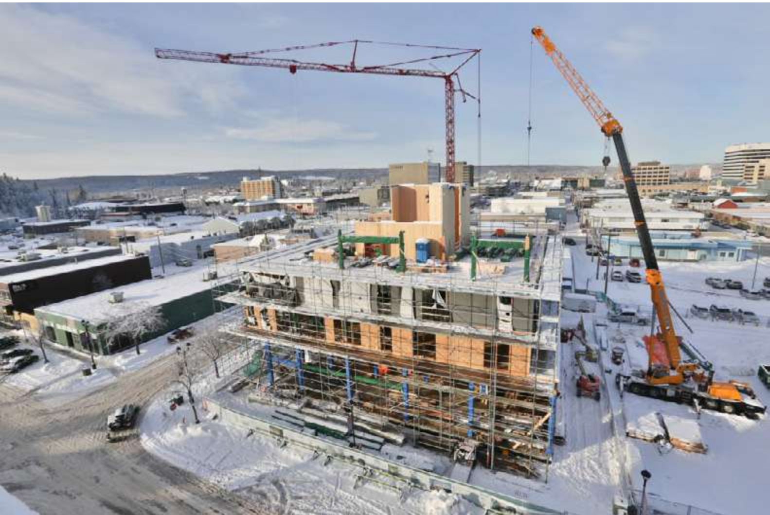
Minimize the number and duration of hoisting equipment rentals. This construction site indicates a variety of cranes, lifts and scaffolding. A generous staging area beside the building and access behind the building allow cranes to work around the entire building without interference. Each project is different and considerable construction experience is needed to optimize the mix of hoisting equipment to efficiently execute the work. (Construction Canada)
