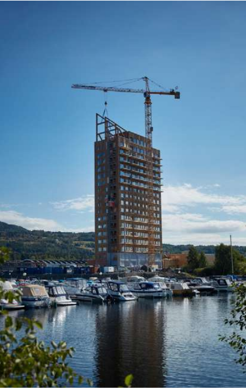
Braced frames avoid the need for shear walls and/or moment connections. Mjøstårnet in Brumunddal, Norway is an 85.4 metre-high tower. At the time of its completion in March 2019, this was the tallest all-timber tower in the world. It does not rely on shear walls or reinforced concrete elevator/stair shafts to resist lateral forces. The Mjøstårnet building’s timber structure consists of a braced frame made from glue laminated timber (glulam) columns, beams and diagonal braces. Floors are not structurally connected to the frame and elevator shafts are made entirely from cross laminated timber (CLT) panels. (Voll Arkitekter)
