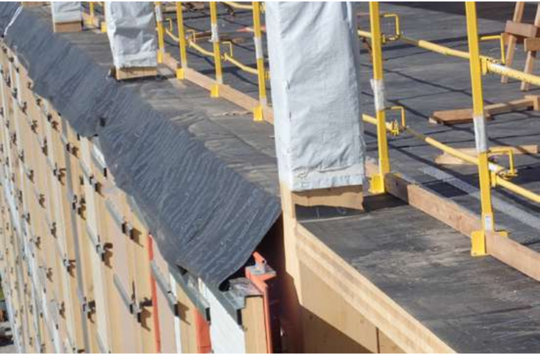
Protective membranes protect CLT floor panels and glulam columns from moisture accumulations. The cost of protective measures must be weighed against the savings due to the reduction in delays caused by bad weather and the elimination of mitigation measures for potential water damage resulting from ineffective moisture management. (Catalyst – Kattera)
