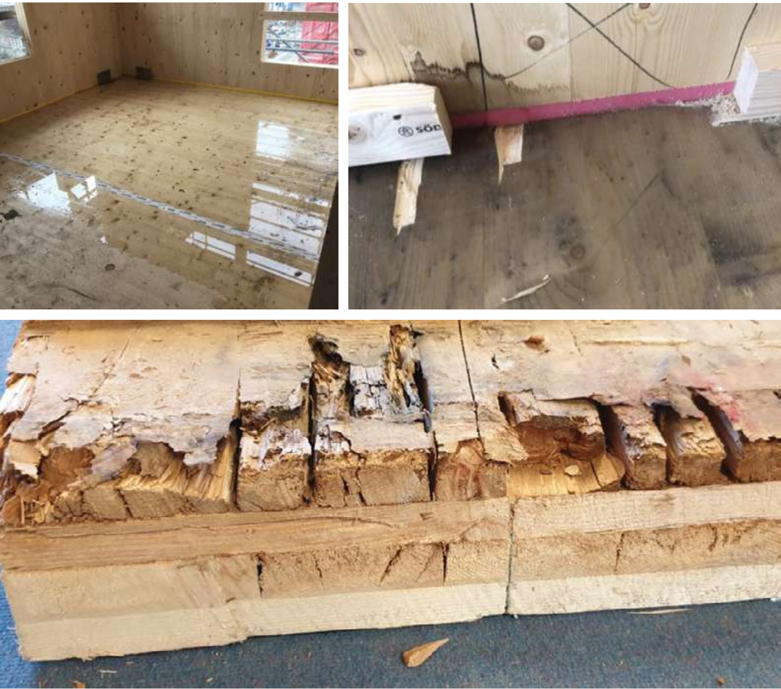
Exceeding the moisture balance of mass timber must be avoided. Moisture absorption for mass timber elements is a delayed process, however, it must be recognized that long-term or frequently recurring exposure to moisture is likely to be more problematic than the overall quantity of water to which the mass timber is exposed. This is because wood absorbs water rapidly and after it is saturated it releases this moisture very slowly as it dries out. In practical terms, trapped and concealed moisture must be avoided by providing multiple layers of defence against moisture intrusion. If the risk of moisture penetration cannot be avoided, then the assembly must be designed so that it is much easier for the water to get out than to get in. The severe deterioration depicted in the lower image occurred in a cantilevered CLT balcony panel suffering concealed moisture migration.
