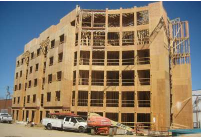
Canadian building codes now permit wood-frame construction up to 6 storeys in height. This has allowed for the relatively economical development of mid-rise multi-unit housing in traditional wood building materials and methods. But now mass timber alternatives to wood-frame offer competitive alternatives with faster erection times. (MFE)
