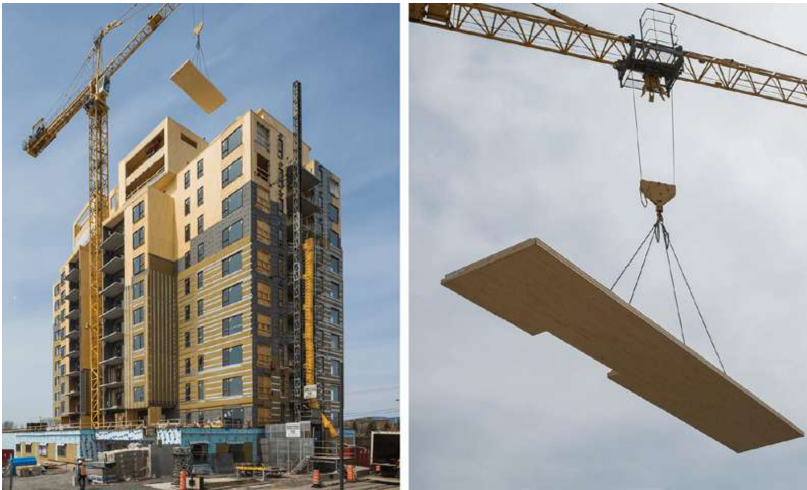
Mass timber panels save construction time. The wooden structure for the Origine project was erected in just four months. It was estimated that about a 25% savings in total project construction time resulted from selecting the mass timber panel structural system. (Cecobois)
