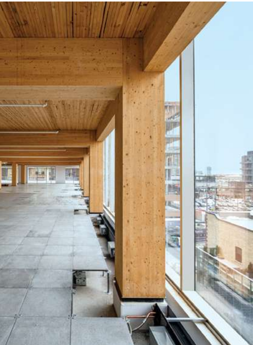
Raised floor systems help address acoustical issues. In addition to helping integrate mechanical, electrical and plumbing systems unobtrusively, raised floor systems, such as this one installed at 80 Atlantic, designed by Quadrangle Architects, also minimize the transmission of airborne and impact sound transmission across floor assemblies. Note that a concrete topping over the NLT floor panels is required to fireproof concealed cavities. (Bob Gundu, Canadian Architect)
