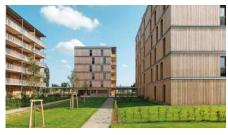
In recent years, wood has become a building material that is increasingly used for innovative projects in urban environments. Thanks to technical advances, it can now be used to implement comprehensive and complex wood structures. This led to the construction of a multi-storey building from MM crosslam cross-laminated timber in the Styrian capital of Graz in 2016.
