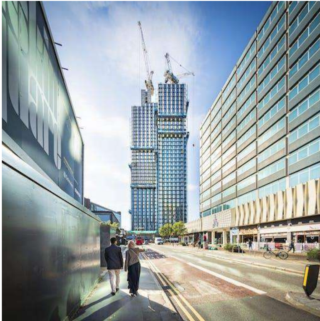
HTA Design's Ten Degrees in Croydon, the world's tallest modular building. Image: HTA Design
