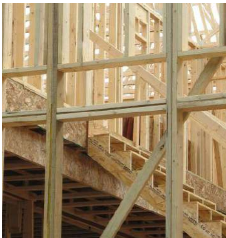
Tomado de: http://www.icanfixupmyhome.com/Residential_Wood_Frame_Construction.html
