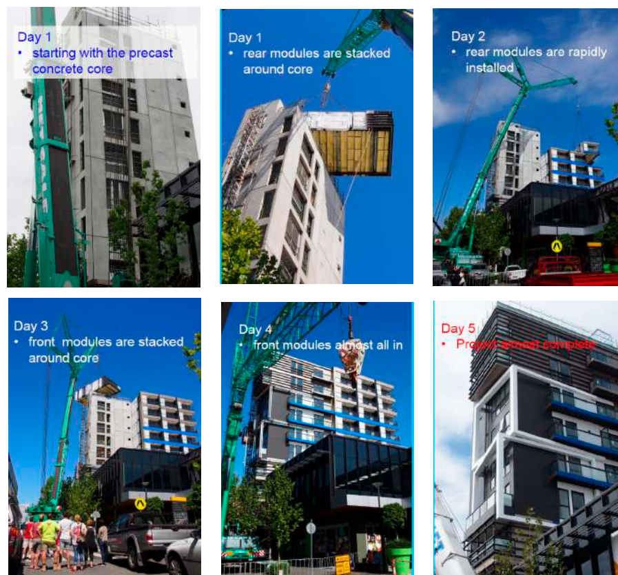
Figure 5. One9 modular building stabilized by a concrete core.
