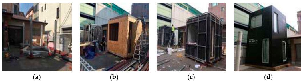
Figure 4. Manufacturing process of flexible modular housing ((a): Installation of columns, (b): Installation of walls, (c) 1F/2F combination, (d) Finished).
