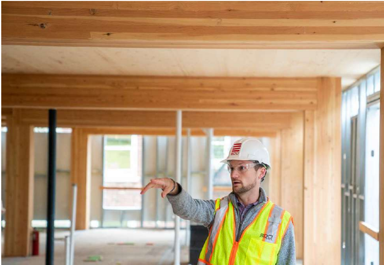
Kevin Miller, DCI project engineer on Heartwood, points out structural highlights on an AIA project tour earlier this year.
