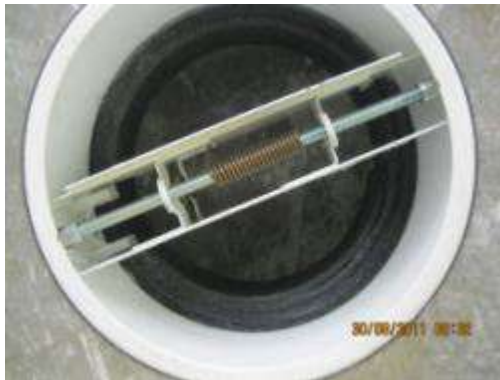
Figure 89: View of a fire protection closure based on intumescent materials with closing element (FLI-VE)
