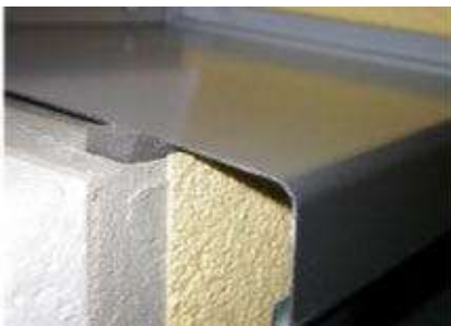
Figure 53: Horizontal joint under window sill towards facade surface with permeable sealing tape. Can also be executed in open form Source: [Österreichische Arbeitsgemeinschaft Fensterbank]
