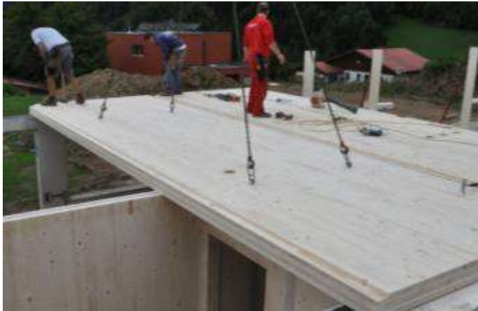
Figure 43: Continuous floors, if used with partition walls, need a suspension in order to prevent sound longitudinal conduction
