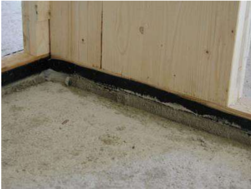
Figure 50: Support detail of an internal wall
