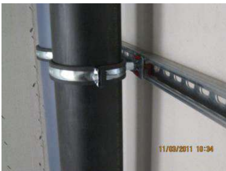
Figure 81: Sound protection decoupling of pipes
