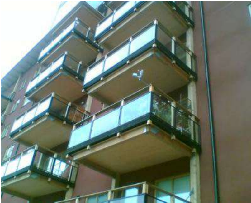
Figure 107: Prefixed balcony construction, source: Stora Enso company
