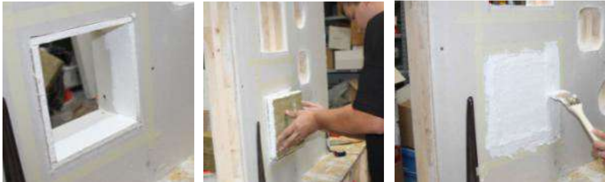
Figure 83: Installation of the soft partition in a sample body (left: reveal covering center: Installation of the mineral fiberboards that is coated on its edges, right: Overcoating of surface beyond the edge of 20mm)
