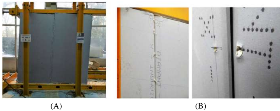
FIGURE 14 Wall collapse. A, Overall deformation. B, Details of the connection failures [Colour figure can be viewed at wileyonlinelibrary.com ]
