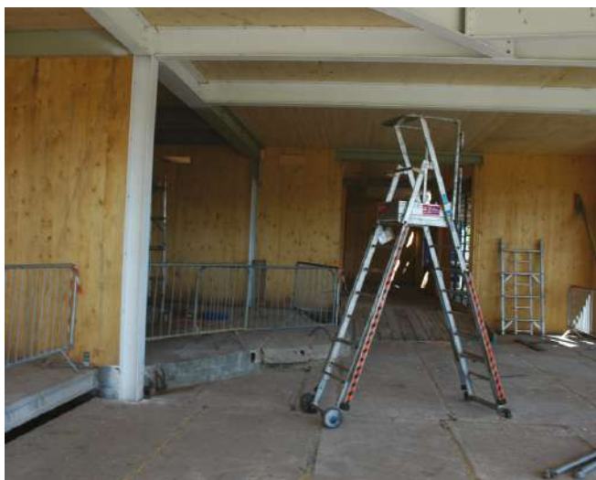
Figure 13 Steel/glulam frame used to support CLT floor
