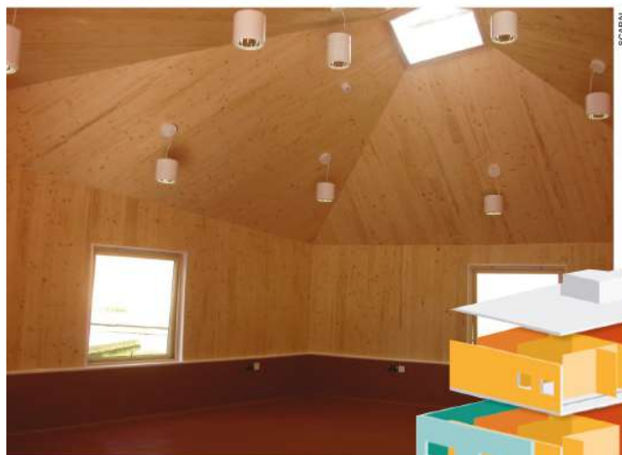
Figure 4 CLT roof panels formed as 'coupled' roof
