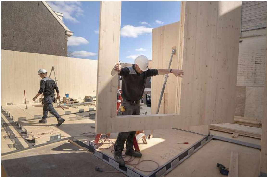
Residential Project, Netherlands
