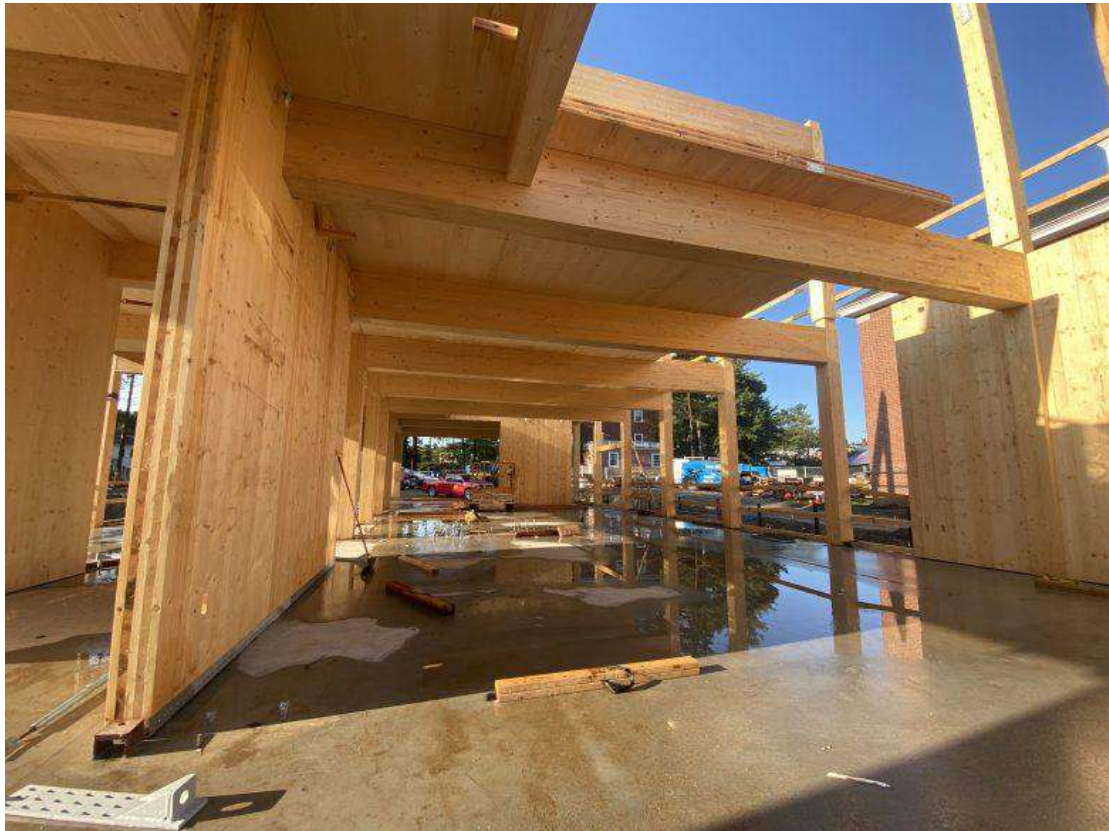
Construction at Bowdoin College using mass timber. Credit: Bowdoin College / Courtesy
