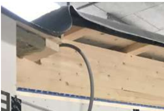
4 Figure 5.5: First layer of roof
