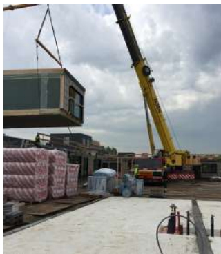
Figure 5.15: Placing on site
