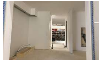
3 Figure 5.4: Interior gypsum plates and paint
