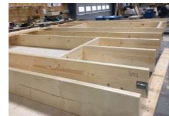
7 Figure 5.8: Second layer of exterior wall
