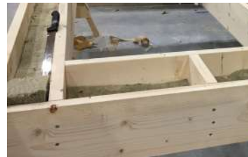
6 Figure 5.7: Insulation on the wall
