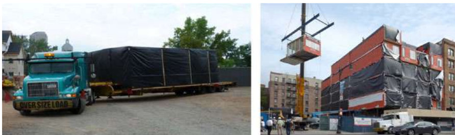
Figure 11. Module transportation and installation. (Image sources: Deluxe Building Systems)
