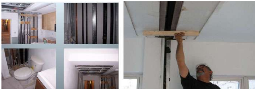
Figure 12. Finishing The Stack. (Image sources: Deluxe Building Systems)
