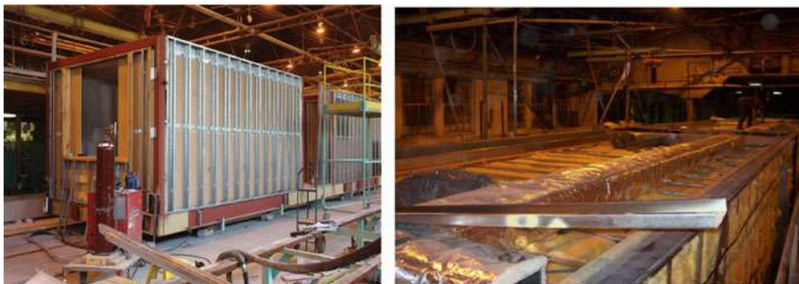
Figure 7. Assembling walls and HVAC ducts. (Image sources: Deluxe Building Systems)
