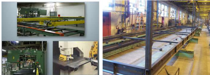
Figure 4. Cutting and assembling a steel chassis. (Image sources: Deluxe Building Systems)
