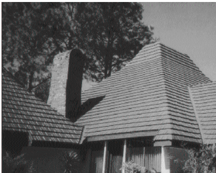
Figure 24: Shingles made from recycled aluminum.
