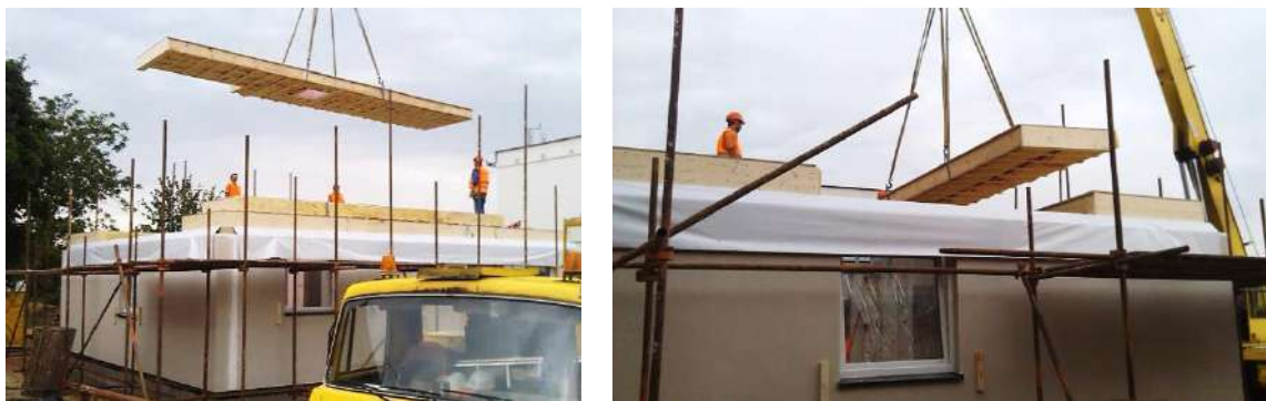
Figure 3. Construction of a prefabricated construction system based on wood.
