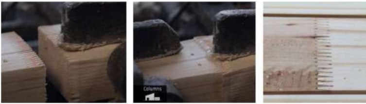
Fig. 2. Finger joint system between CLT panels (Cree Buildings, 2015; Crosslam, n.d.)
