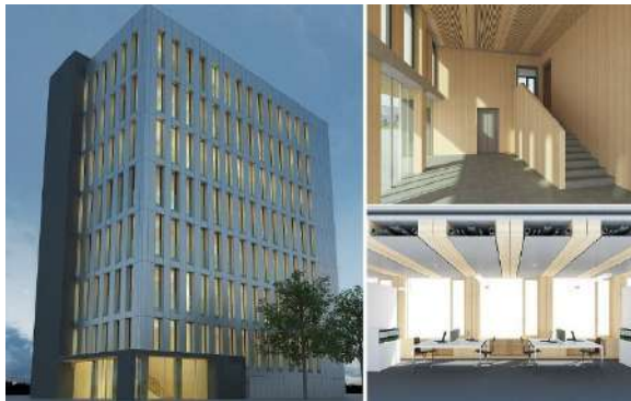
Fig. 5. Lct One building (Gayle, 2012)
