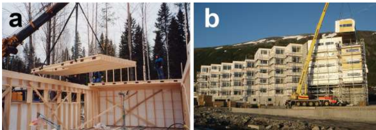
Figure 1.11 Prefabricated elements and modules: a) Prefabricated mass timber floor in Northern Sweden, late 1990s (Photo Martin Gustafsson), (b) Modular houses in Norway (Photo Kodumaja).
