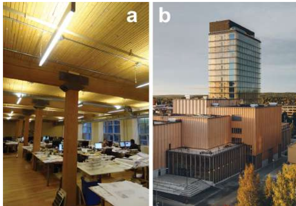
Figure 1.8 Mass timber panels construction: (a) Old mill floor in Canada (Photo FPIInnovations); (b) Sara Cultural Centre and hotel, 19 storeys, Skellefteå, Sweden (Photo Jonas Westling).
