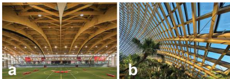
Figure 1.9 Long-span timber systems: (a) Soccer stadium in Canada (67.6 m span) (Photo Nordic Structures © Stéphane Groleau), (b) Timber grid shells in China (43 to 88 m span) (Photo StructureCraft).
