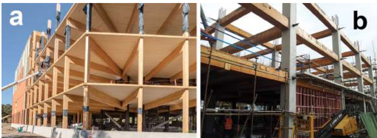
Figure 1.2 Office buildings using timber product: (a) First Tech Credit Union office in Canada (photo Structurlam Mass Timber Corp.); (b) Hybrid office building in New Zealand (photo A. Buchanan)
