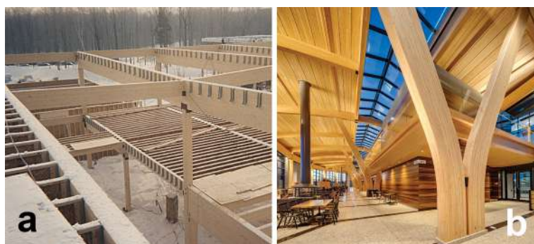
Figure 1.15 Structural glued laminated timber: (a) Post-and-beam construction using glulam and prefabricated wood I-joists (photo FPIInnovations); (b) Curved beams and decking at ATCO commercial centre in Canada (photo Western Archrib).
