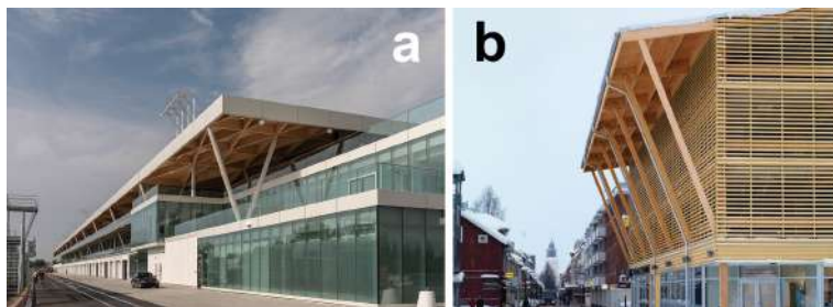
Figure 1.4 Public buildings using timber products: (a) Formula 1 paddocks in Canada (Photo Nordic Structures); (b) Parking garage in Sweden (Photo AIX Architects).
